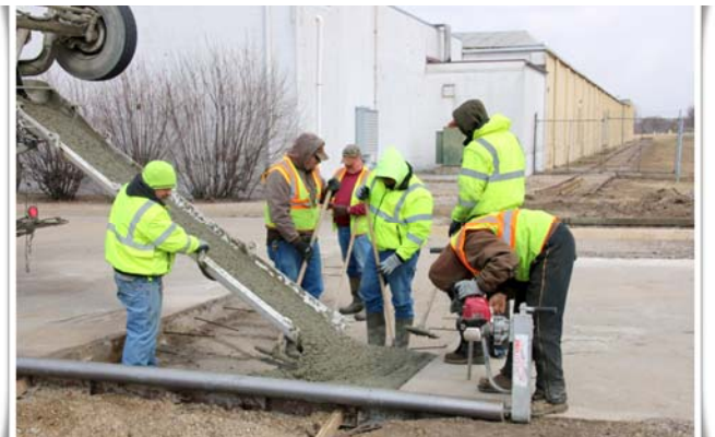
Street Improvements on Boulevard St.
